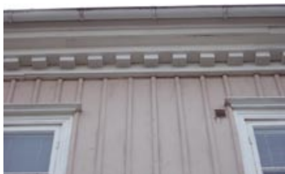
Fasaddetalj under takfoten
